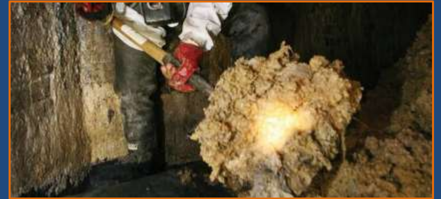
London Sewer System Cleaning
