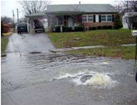
Sanitary sewer manhole overflow
