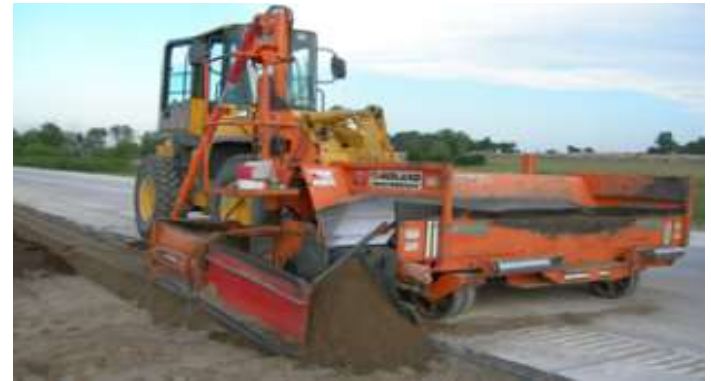
Use of recycled concrete and asphalt in highway construction
